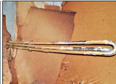
The view into the inside of DHW storage tank after the partial encrust removing.
